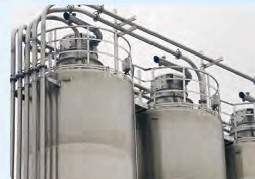
储料仓 Storage Silo
